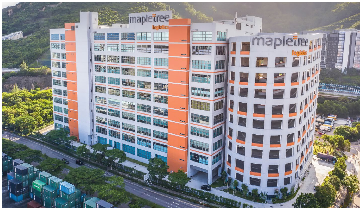
Mapletree Logistics Hub Tsing Yi
