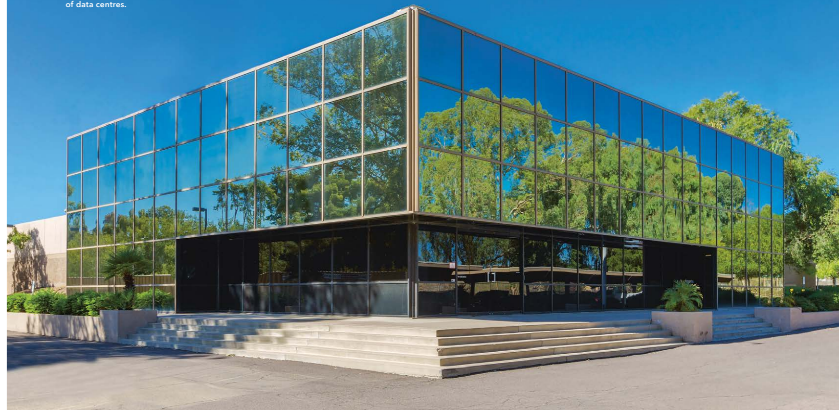
2601 West Broadway Road, Tempe located in Arizona, the US, is part of the Group’s growing portfolio of data centres.
