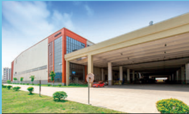
Mapletree Wuxi New District Logistics Park
