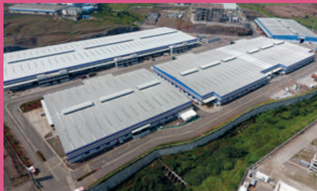
Mapletree Logistics Trust India KSH Industrial Park 1
