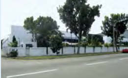
44 44 & 46 Changi South Street 1
