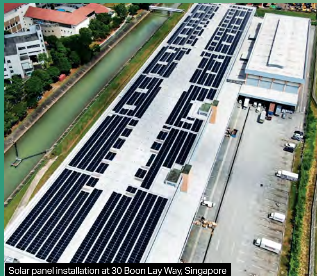
Solar panel installation at 30 Boon Lay Way, Singapore
