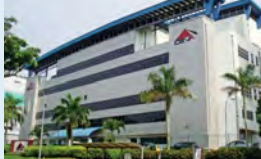
40 15 Changi South Street 2
