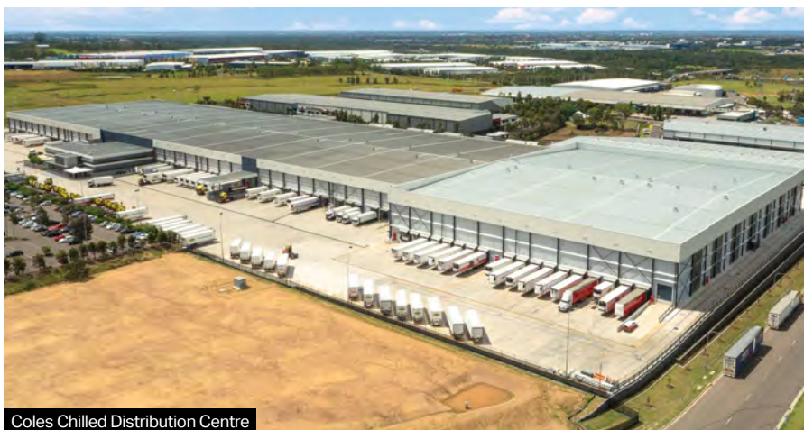
Coles Chilled Distribution Centre
