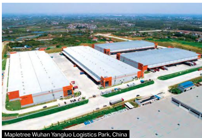
Mapletree Wuhan Yangluo Logistics Park, China
