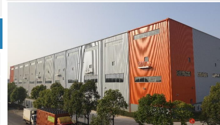
Mapletree Ouluo Logistics Park, Phase 1
