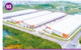
93 Mapletree Changsha Logistics Park Phase 1
