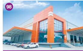
98 Chengdu DC Logistics Park
