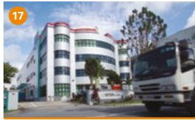
17 39 Changi South Avenue 2
