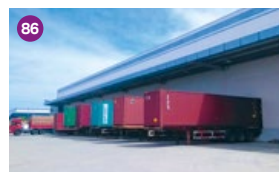
Mapletree Yangshan Bonded Logistics Warehouses
