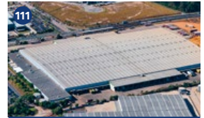
111. Coles Brisbane Distribution Centre, 44 Stradbroke Street, Heathwood, QLD (formerly known as Coles Brisbane Distribution Centre, QLD)
