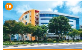
19 10 Changi South Street 3
