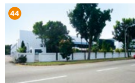
44 44 & 46 Changi South Street 1
