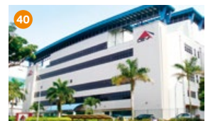
40 15 Changi South Street 2
