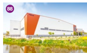
Mapletree Wuxi New District Logistics Park
