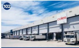
102. Coles Chilled Distribution Centre, NSW
