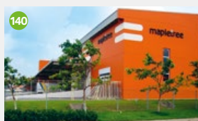
Mapletree Logistics Centre
