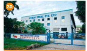
30 31 & 33 Pioneer Road North (formerly known as Union Steel (Pioneer))
